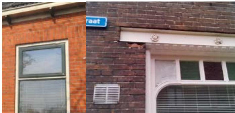
Figure 2.1. Type of lintels. Masonry lintel (left) and steel lintel (right).
